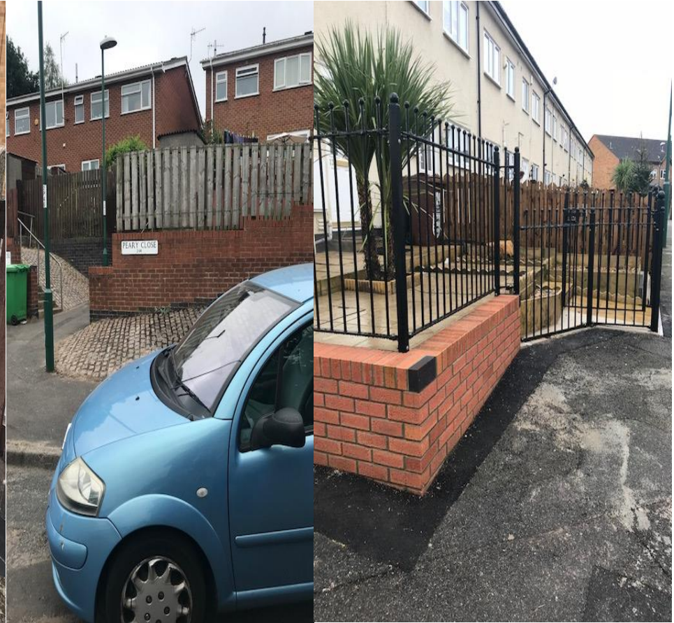
Example of new railings on brick wall
